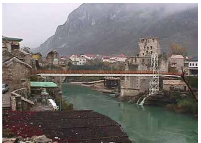
WiRED installed four MICs here in Mostar, Bosnia. Mostar was once a frontier town of Ottoman Empire.
